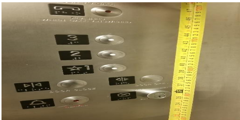
Elevator buttons are low enough to accommodate a person in a wheelchair. (36”)
